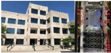
Data Center Durham Center, ISU
