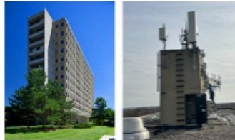
Base Station Wilson Hall, ISU
